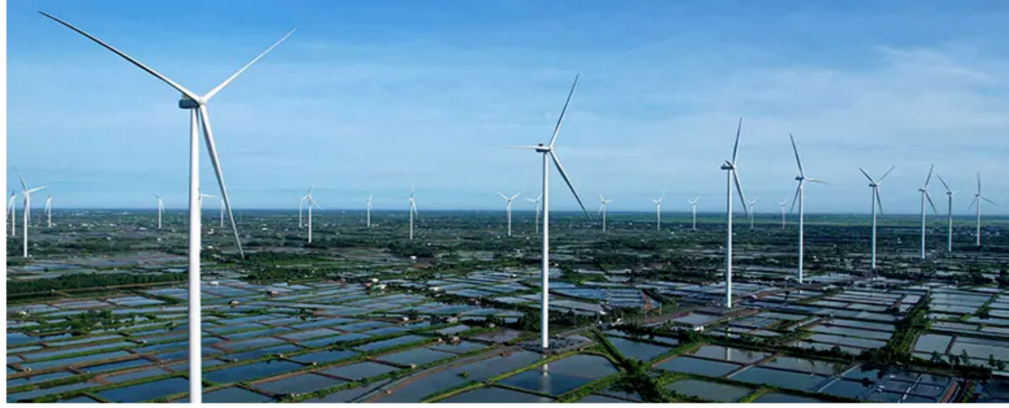
A group of wind turbines in a rice field
